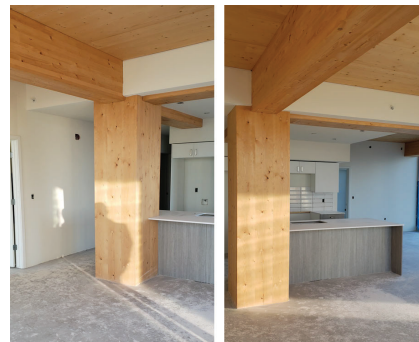
Figure 1: Interior views of exposed mass timber framing (Ascent building, Milwaukee, Wisconsin – USA). Photo © David Barber.
