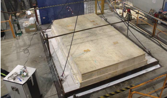
Figure 1: The floor specimen mounted on the horizontal furnace (Photo: RISE Fire Research AS)
