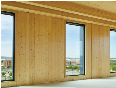
Figure 2: Five story building constructed in the US with CLT exterior wall approved without NFPA 285 fire testing (image credit: Blomgren)
