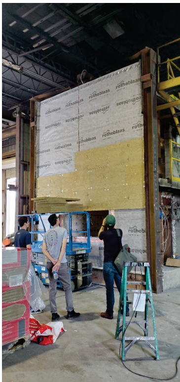
Figure 9: Test 1 set up, showing installation of mineral wool (image credit: Barber)
