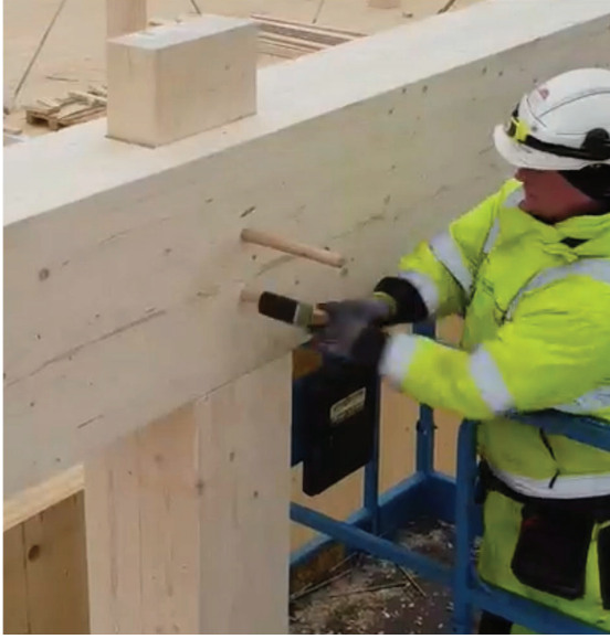
Figure 6: Hardwood dowels during assembly of timber structure.
