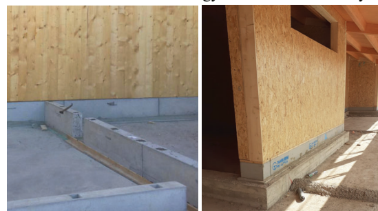
Figure 1: Prefabricated concrete beam-foundation element example of use on construction-site (CLT and LFT walls)
