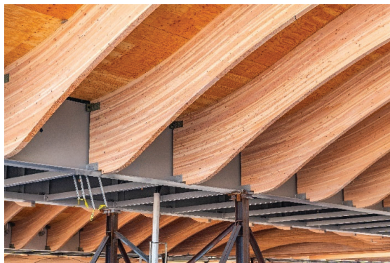
Photo 1: As constructed glulam beam end moment connections
