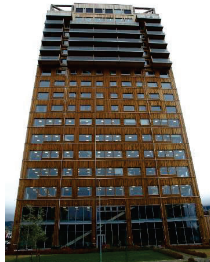
Figure 1: Mjøstårnet in Norway, 18 story glulam building.
