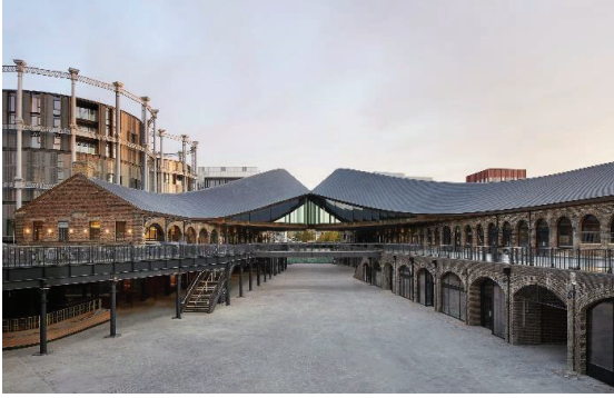
Figure 5: Coal Drops Yard, London (© Hufton Crow)
