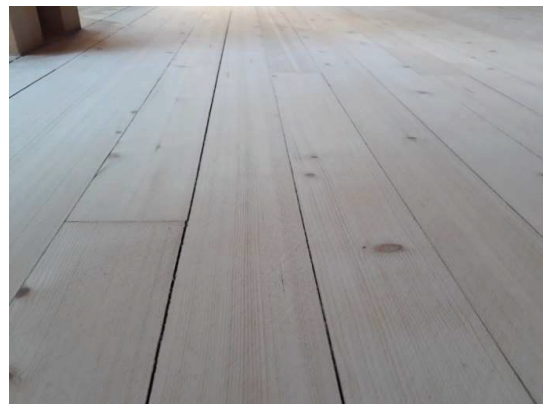
Figure 11: The floor after it had been sanded the first time after fifteen years. If the floor will be sanded regularly, it is impossible that the surface would start to patinate as the old wooden floor. On the other hand also the used dimensions are smaller than in the past.
