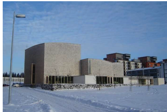
Figure 5: Viikki Church in winter 2006. The exterior of Viikki church is clad in cleft aspen shingles and they have turn grey during time as originally planned.
