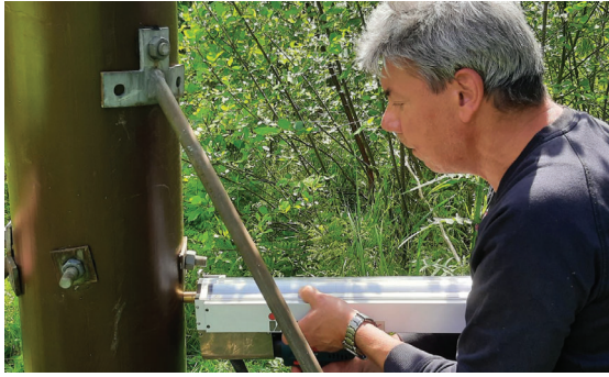
Figure 5 Drilling measurement using a resistograph, close to pin bolt with curved washer and mastic.
