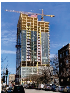
Figure 1: Ascent (Photo courtesy of Thornton Tomasetti)
